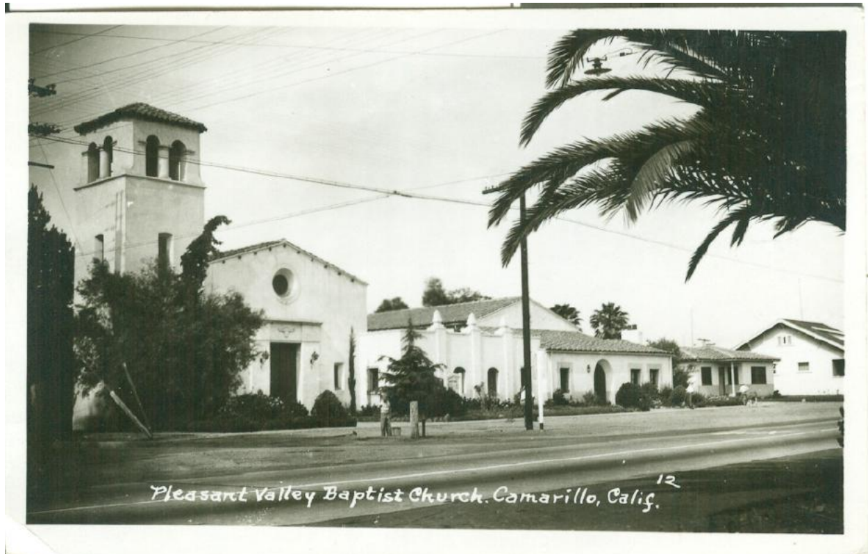
Pleasant Valley Baptist Church was dedicated August 10, 1930. Harold Burket, son-in-law of Adolfo Camarillo, was the architect.
