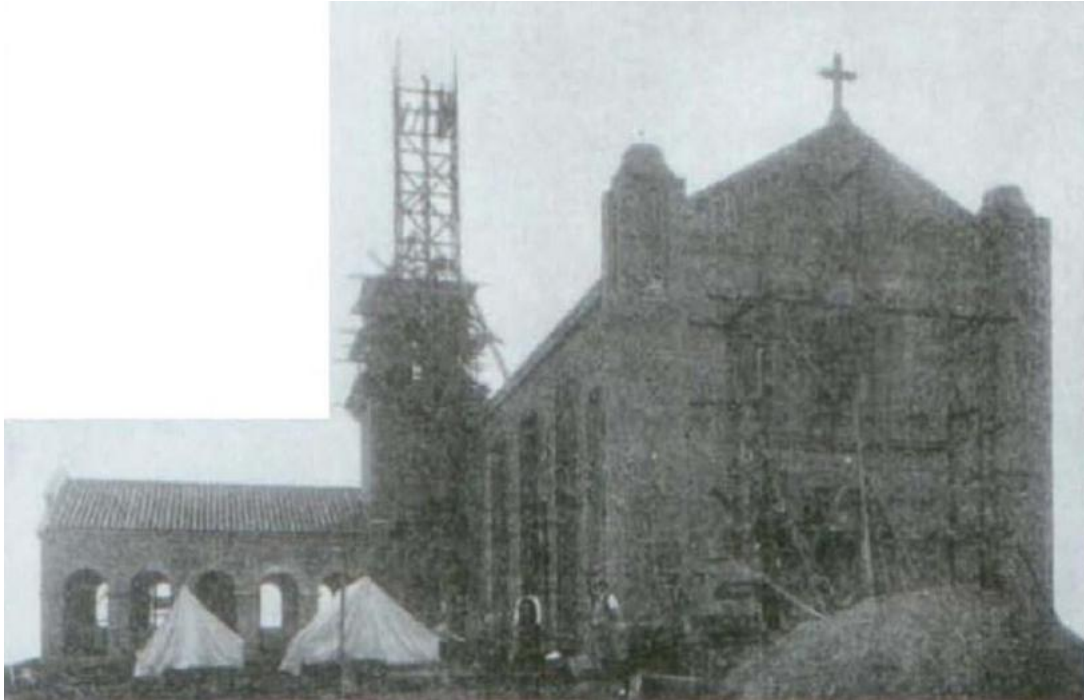
Chapel under construction
