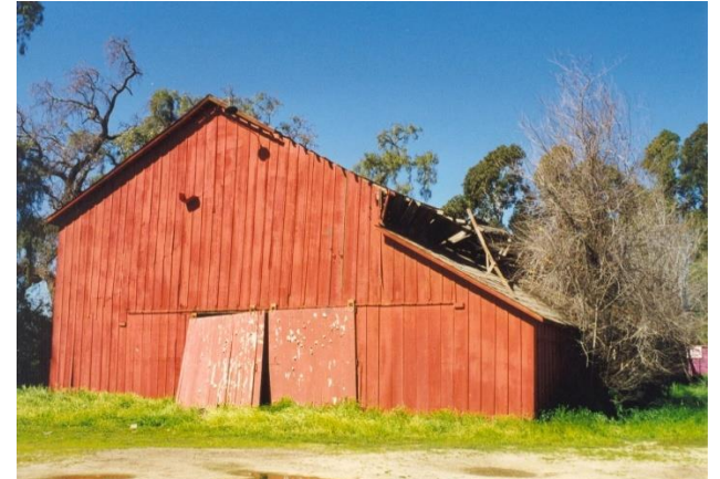
South side of Carriage Barn/Walnut Processing Bldg.
