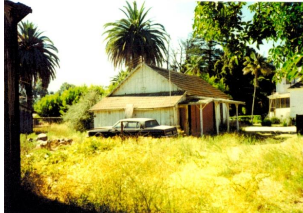
West Storage Building (Ranch House at right)
