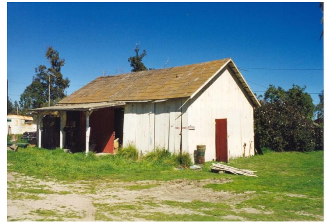
West Storage Bldg. (red door faces Ranch House)
